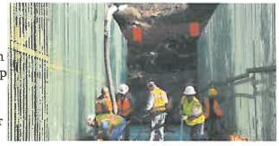
the railroad tracks! The installation of the freeze pipes at the north portal is getting close to completion. In about two weeks, all the freeze pipes will be in place and the freezing process can begin. That will take about 4
